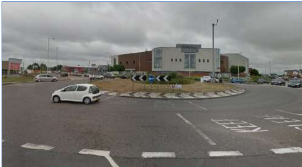
Figure 4 - Westwood Roundabout (A256/A254)
