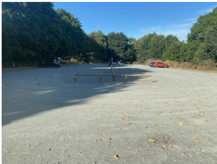
Teston Bridge overflow car park following resurfacing
