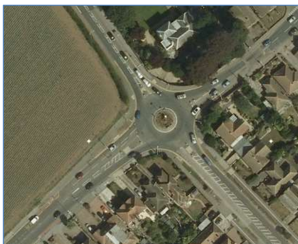
Figure 16 - A256 / A255 Dane Court Roundabout
